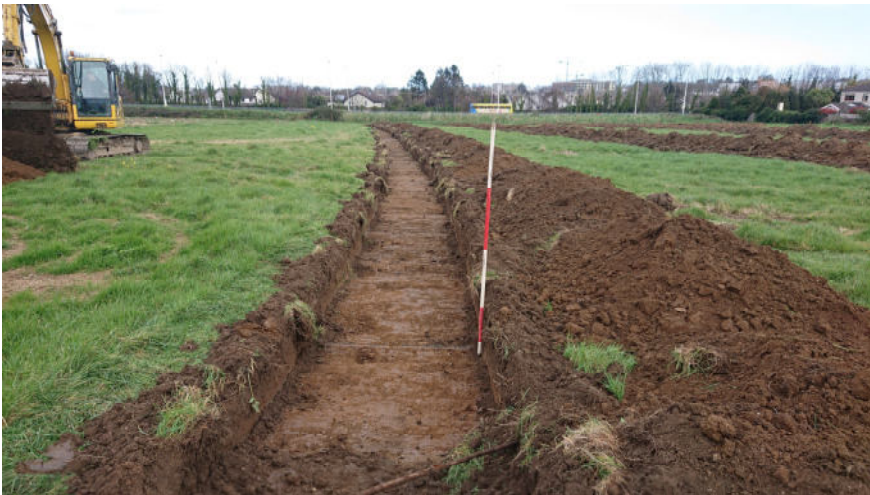
Plate 10: Trench 5 looking north-east
