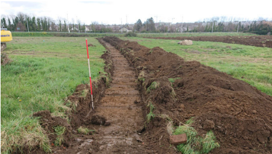
Plate 12: Trench 7 looking north-east
